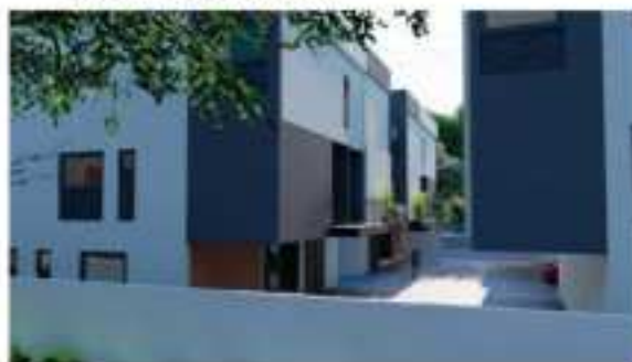
BOTH BLDG - SIDE VIEW
