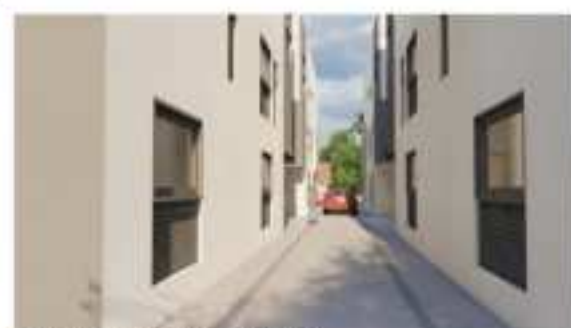
BLDG 3&4 - IN BETWEEN VIEW
