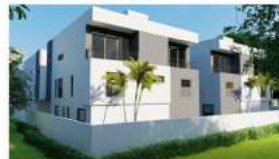
REAR BLDG - REAR VIEW
